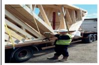
7. Once the pack is supported the driver can assist the responsible person by cutting the rope attaching the pack to the bars. This must be carried out from a safe position using the drivers cutting tool.
