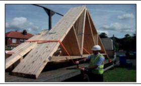
Ensuring the blue rope is holding the outer pack the driver will cut the yellow banding to allow separation of the individual trusses.
