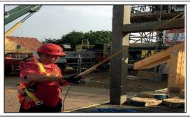
8. The driver will untie the blue rope then separate the 1st truss at the heel by hand or use of crowbar then replace the rope around the remaining trusses, repeating this process at the other end of the truss ensuring that, at all times, there is at least one rope securing the remaining trusses in the pack back to the centre bars.
