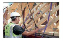
5. Once the order of unloading is agreed between the slinger and driver, the slinger will attach the purple lifting slings to the crane hooks
