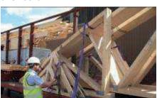
**3**. The manufacturer will supply truss packs secured to the trailer with 8mm blue rope. You should familiarise yourself with which rope attaches which pack to the centre bars.
