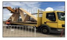
**6.** When instructed that the area is clear the FLT Operator shall remove the trusses from the lorry.
